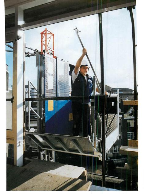
Electrically interlocked fold down ramp.
