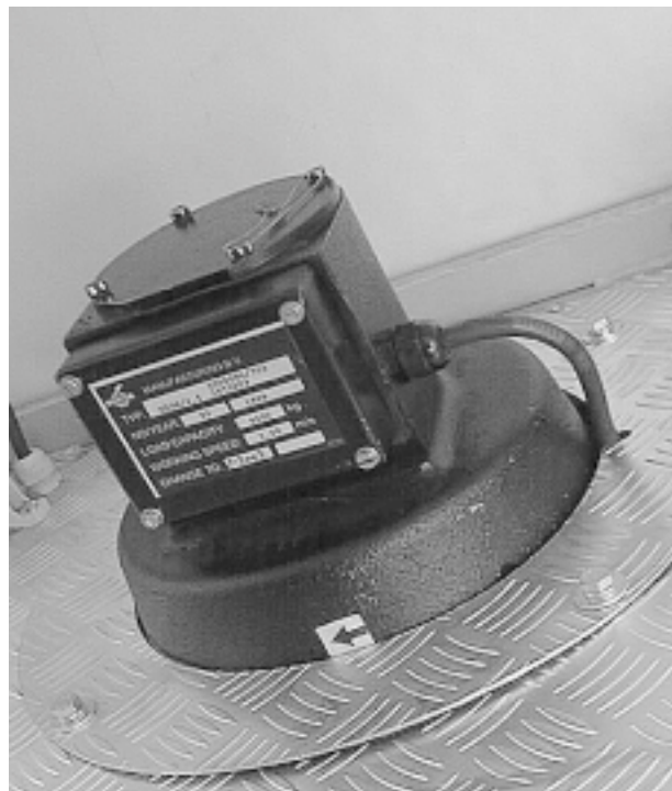
Fig. 7-5 Failsafe brake
